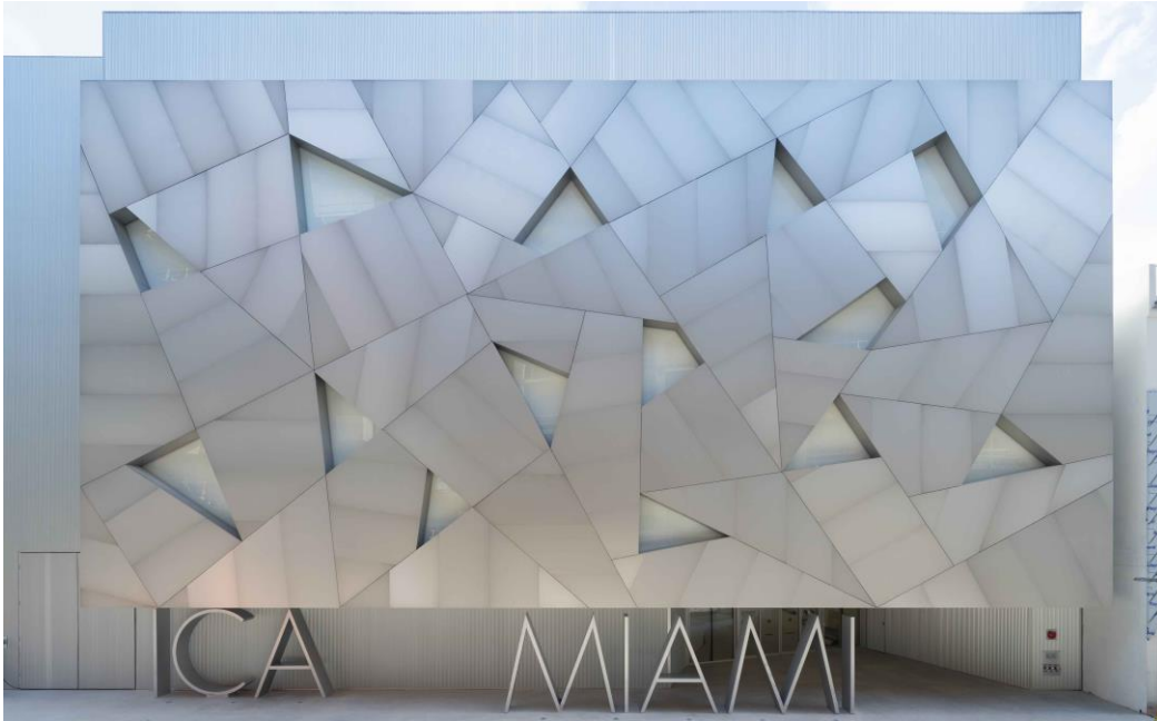
Photo of new ICA Miami's exterior. Image courtesy Iwan Baan.
